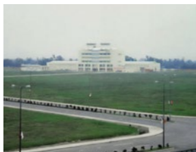
Vietnam Factory at founding
