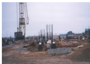
Vietnam Factory at the time of construction
